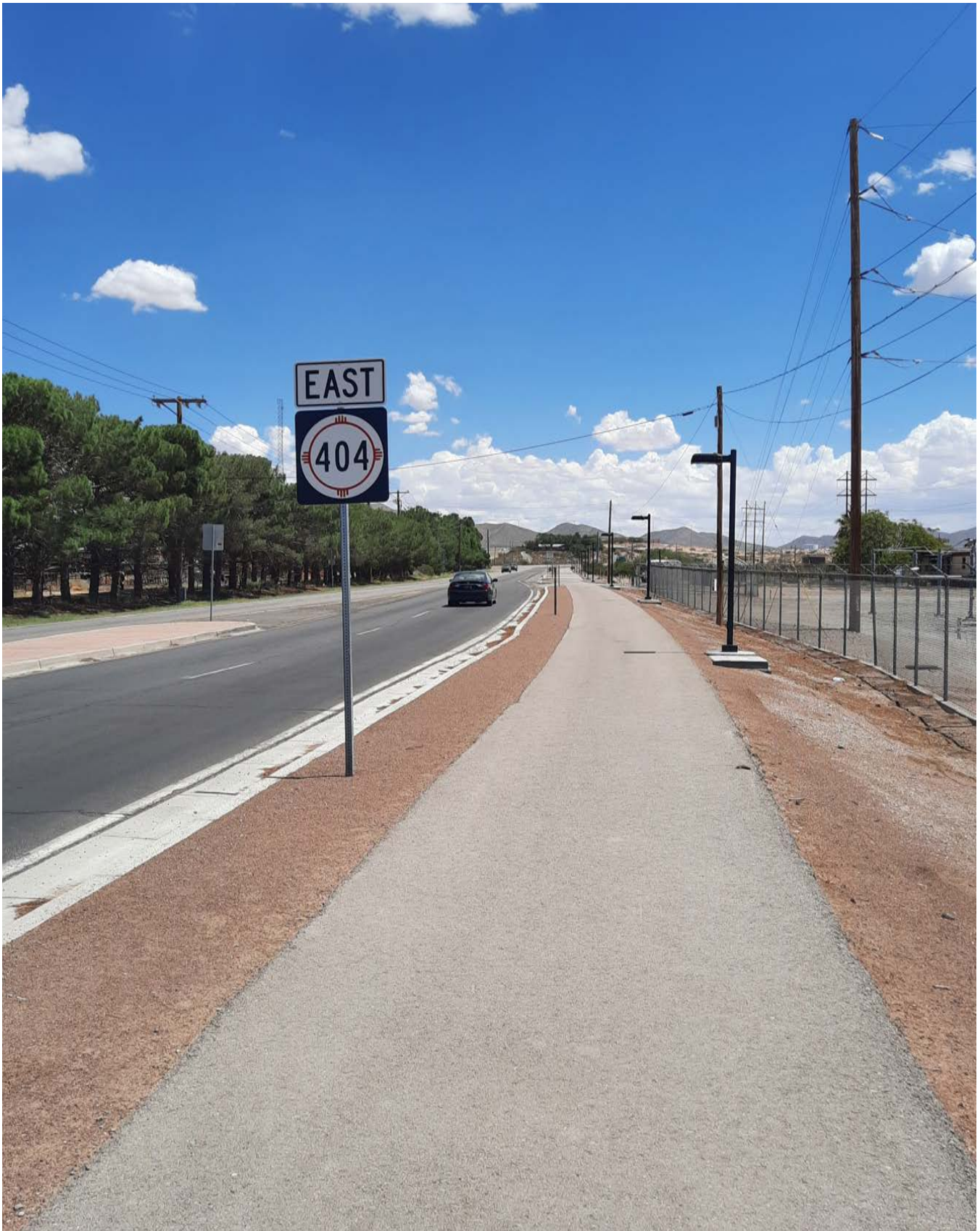
PAVED MULTI-USE TRAIL ALONG OHARA ROAD (NM 404) IN ANTHONY, NM. THE TRAIL IS LOCATED AT CURB LEVEL AND TAKES THE PLACE OF A SIDEWALK.
