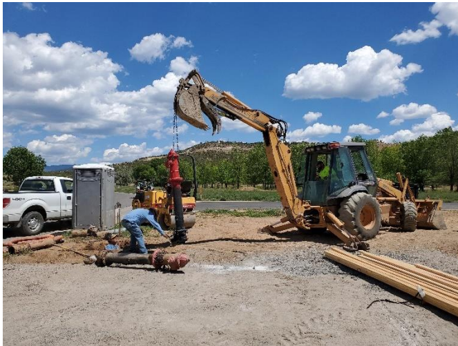
Figure 12: Fire Hydrant Installation (Source: Town of Cedaredge)
