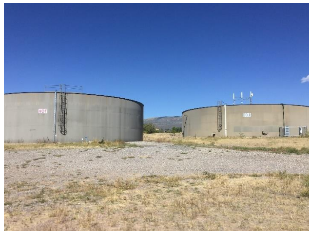
Figure 13 Town Water Tanks (Source: Town of Cedaredge)
